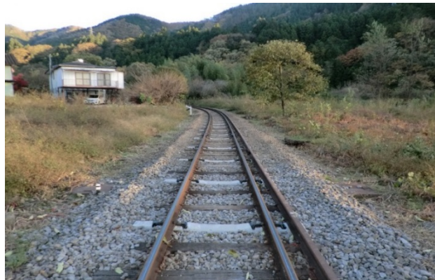
Figure 8. Example of partly changed PC sleepers
